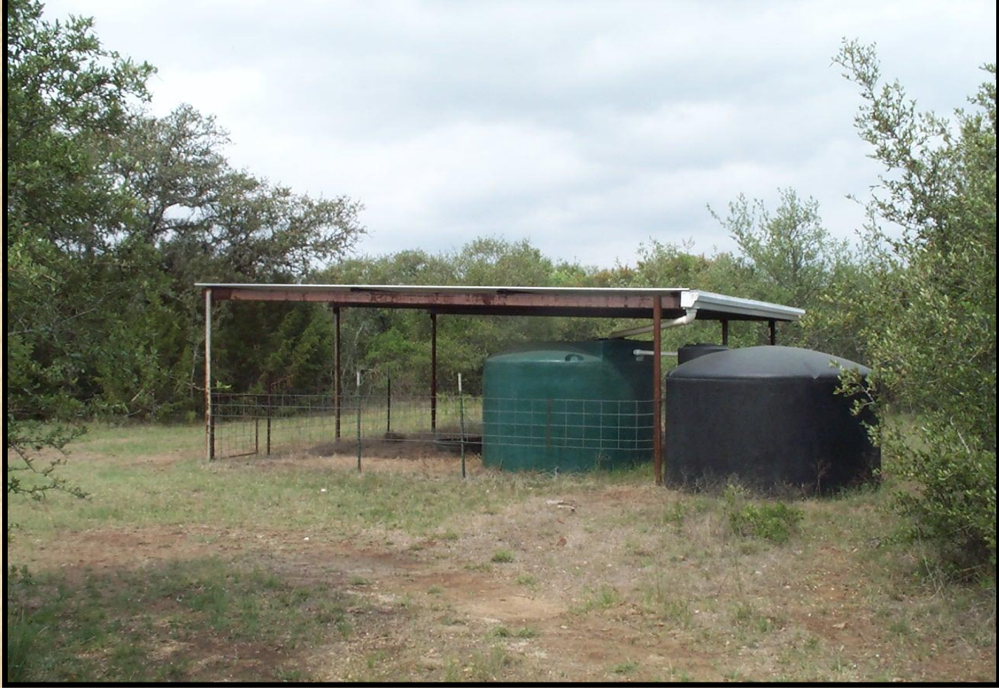
Texas State University's Freeman Ranch Wildlife Water Guzzler – 20' x 20' Roof And Two 1500 Gal. Tanks. The Fence Keeps Livestock Out.
