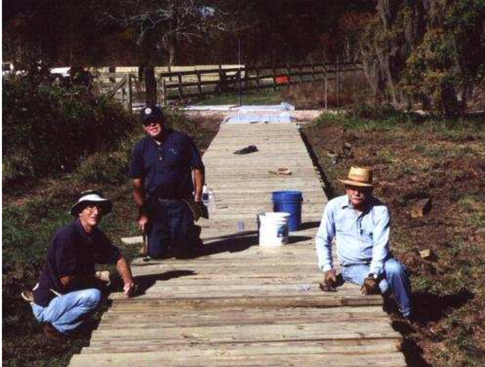
Boardwalk Construction. Photo by Jerry Krampota, 2004.
