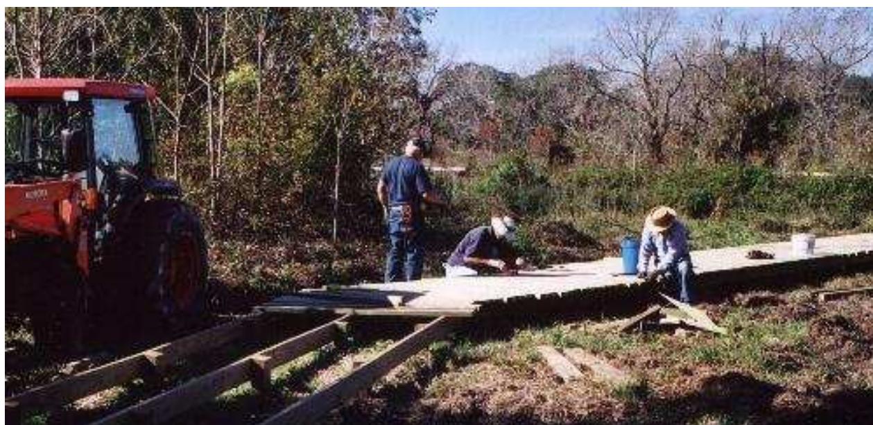
Boardwalk Construction. Photo by Jerry Krampota, 2004.
