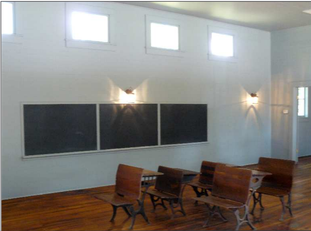
Interior of the Columbia Rosenwald School during renovation, looking northwest, August 2009. Note the small windows above the blackboards on the west side of the building.
