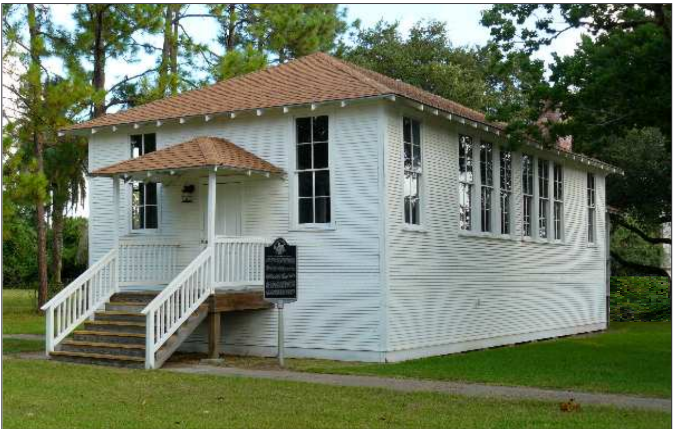
Columbia Rosenwald School during restoration West Columbia, Texas, August 2009
