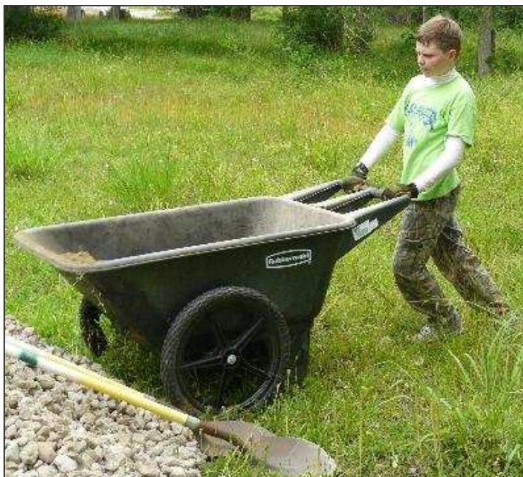
Aaron Sanchez , back for another load of crushed concrete.
