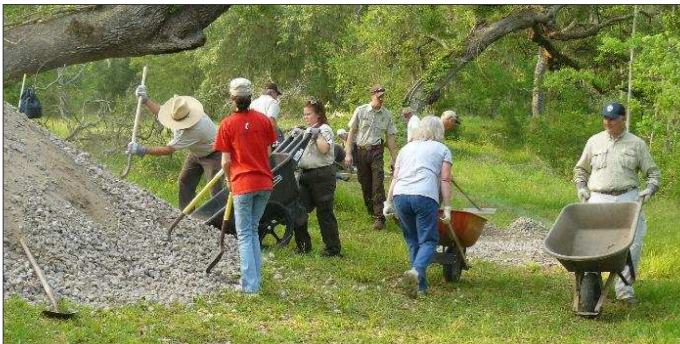
Hauling crushed concrete.
