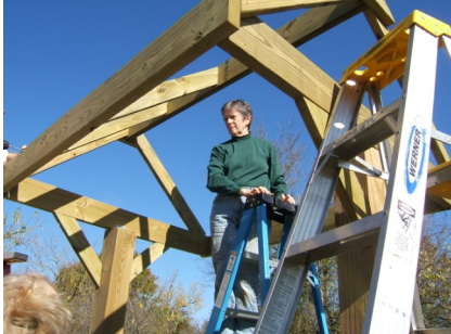
Building is part of MN volunteering —Peg La Point working on kiosk at Clear Creek (photo Jan Thompson)
