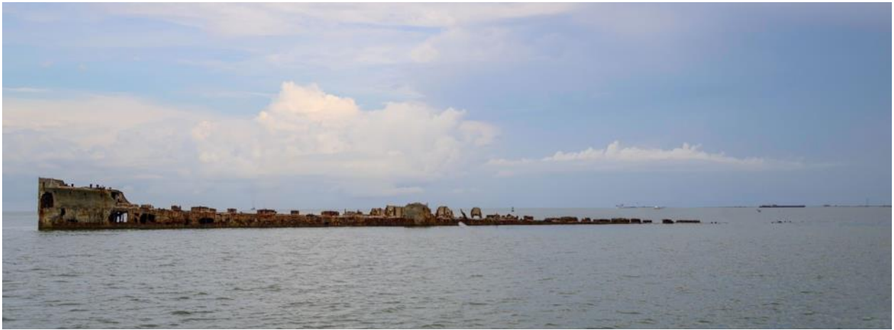
Above: S. S. Selma, WW I Concrete Vessel off Pelican Island Below: Selma Close up
