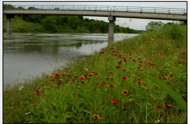
RR outflow channel
