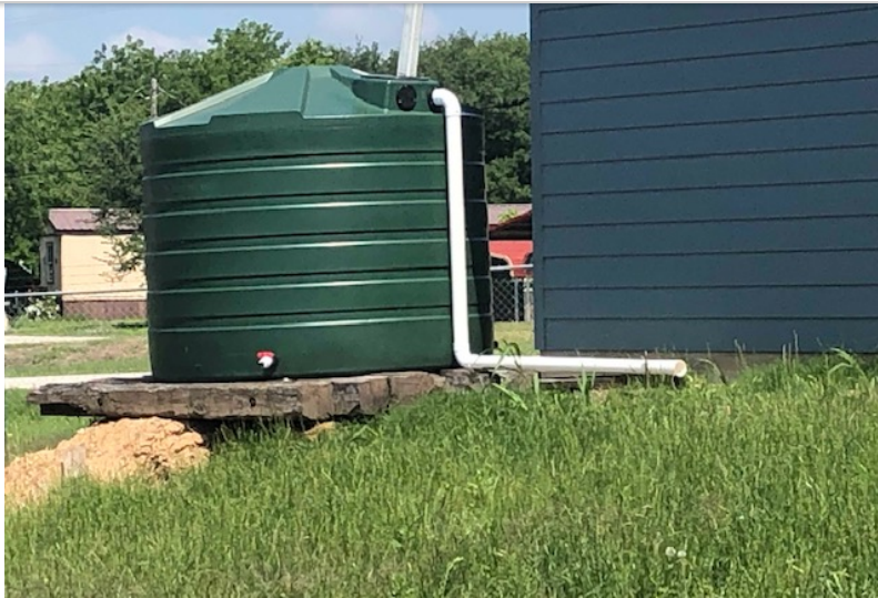
The museum installed a rain capture system to supply a source of water.
