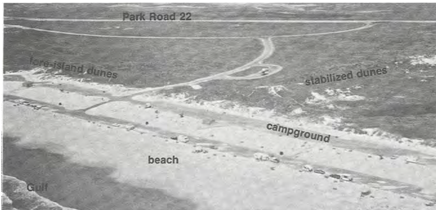
Figure 8. Paved campground just north of Malaquite Beach visitor facilities. The campground, located on the backbeach, was extensively damaged during Hurricane Allen in August 1980 (see p. 73). The above photograph was taken before the storm.
