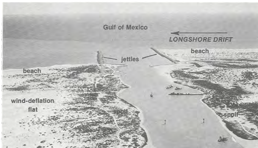
Figure 13. Mansfield Channel (pl. I, grid C-21). This channel, dredged through the island and lagoon in 1957, is used heavily by shrimp boats. The two jetties, constructed of large granite blocks, keep the channel mouth from being filled with sand transported by longshore currents, which generally move from south to north (right to left) here. View is to the east.
