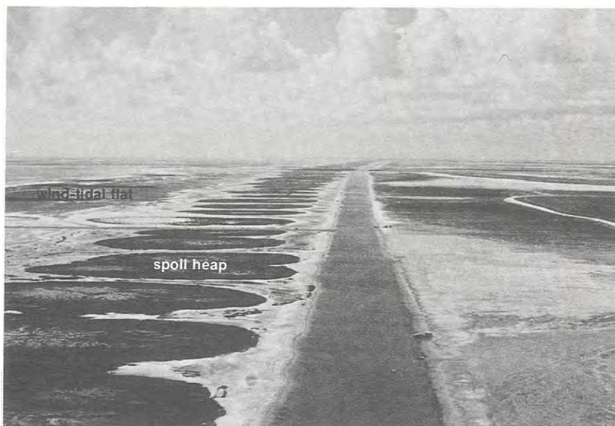
Figure 11. Intracoastal Waterway, approximately 12 feet deep, paralleled by a row of spoil heaps (pl. I, grids P-7 and Q-7). In this area the boundary of the National Seashore does not coincide with the Waterway but rather lies farther to the east (left). View is to the south.
