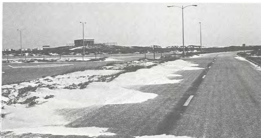
Figure 69. Tongues of sand blown by onshore winds onto a road near Malaquite Beach. Gulf is to the left.
