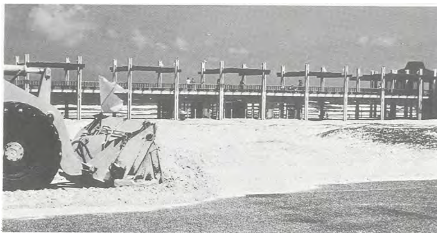
Figure 68. Bulldozer scraping windblown sand off the paved parking lot at Malaquite Beach. View is gulfward.
