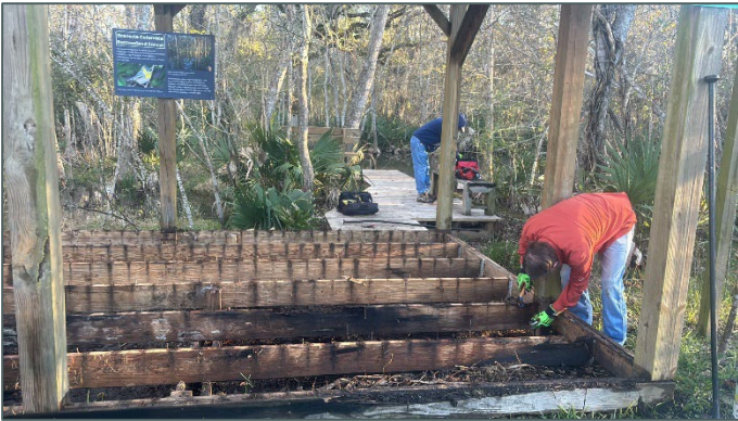
Replaced rotted deck on the birding tower at Gulf Coast Bird Observatory. Work Crew: Robin Townsend, George Valadez, Dick Schaffhausen, Tom Taroni, Oron Atkins
